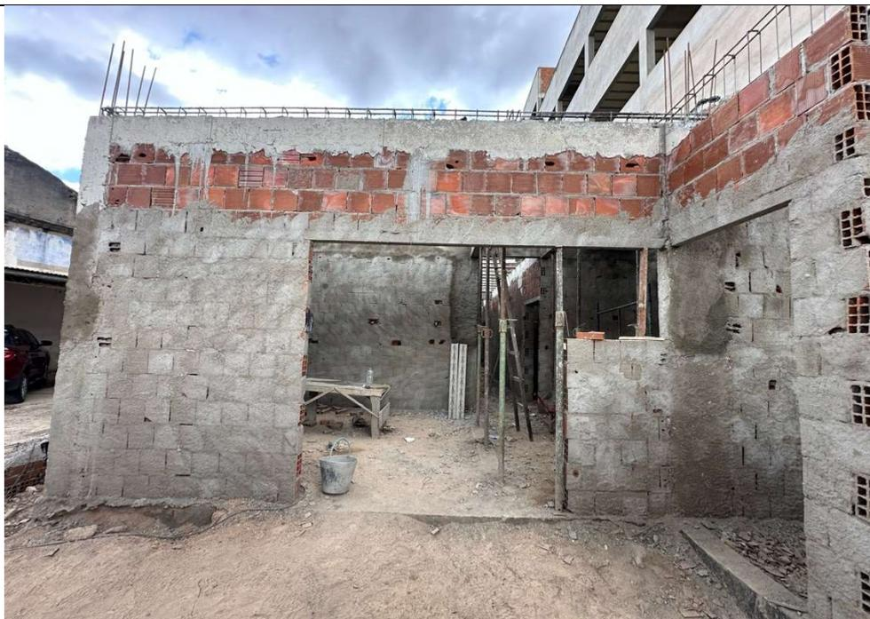
**FOTO 05 – VIGAS CONCRETADAS/CHAPISCO**
