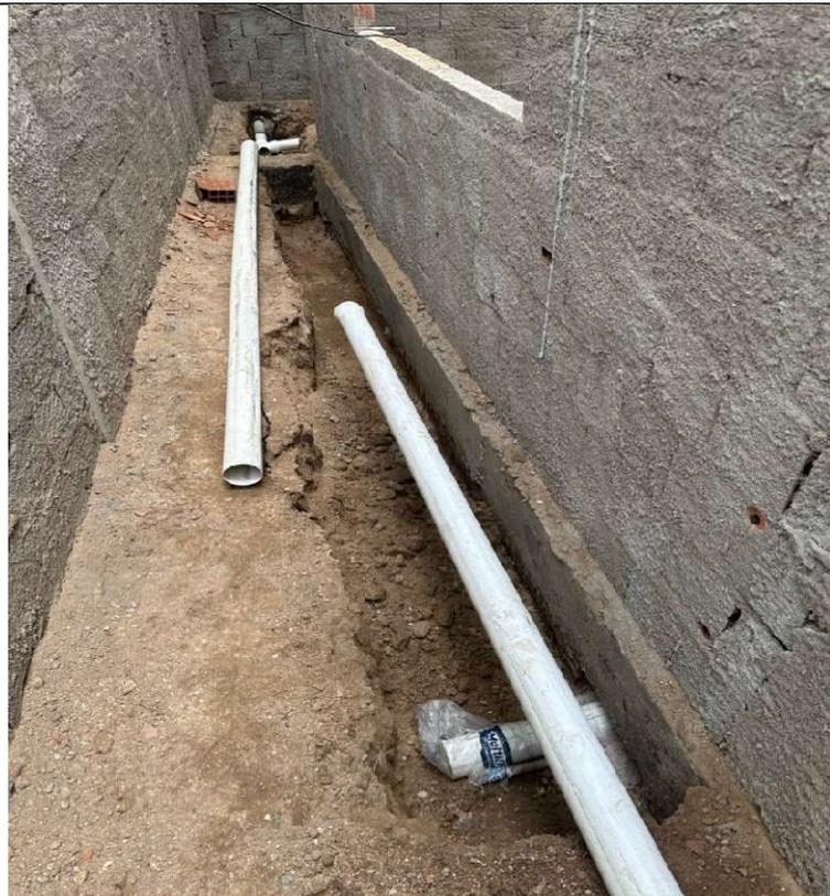
**DETALHE: INSTALAÇÕES SANITÁRIAS EXTERNA**
